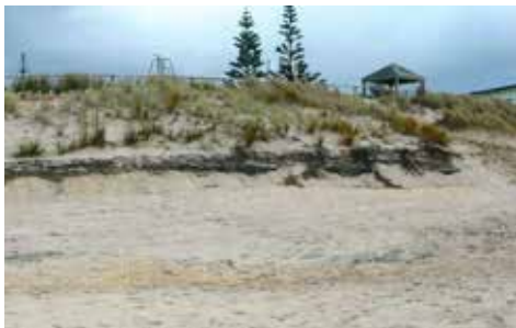
Erosion in the central areas of the beach is causing concern.
