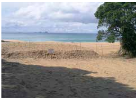
The small dune constructed to intercept windblown sand that had been causing issues for properties neighbouring the beach.
