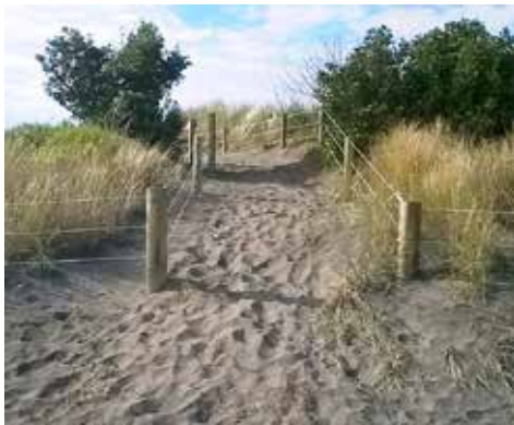
The realigned beach access way at Te Kopua protects the dune plantings and is more successful than the original access way that was suffering from wind erosion during strong north west winds.
