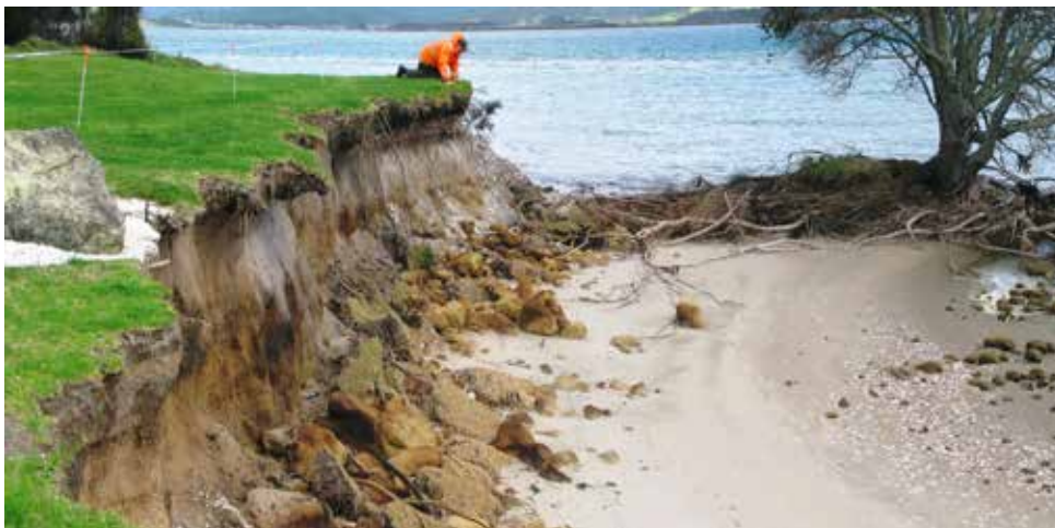
The erosion at the Matarangi Spit near the harbour entrance.
